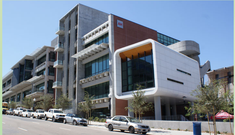
Arts and Humanities Building
