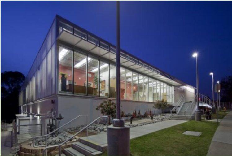
“P” Building Renovation
