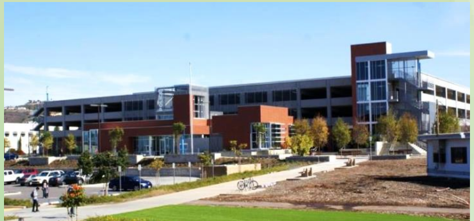
Police Station & Parking Structure
